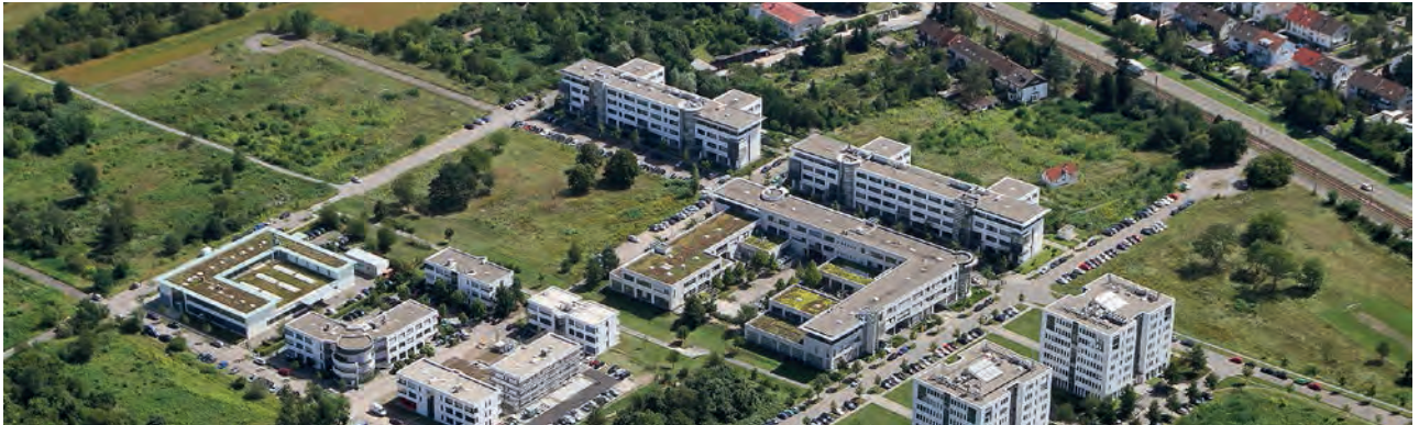
Existing technology park and Rhine dock cluster, Image: Roland Fränkle, Press and Information Office
